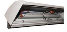
5. Hook luminaires onto wall plate tabs.
