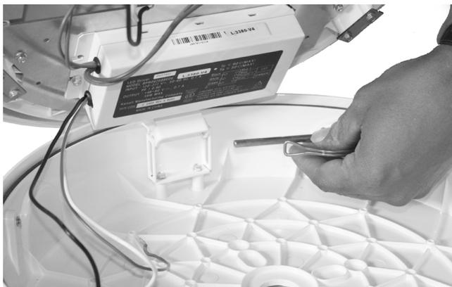
3. Set luminaire on donut to protect sensor while installing housing.
