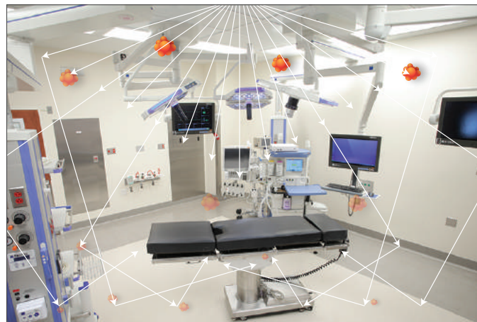
White disinfection mode provides ambient lighting and continuous environmental disinfection while occupied
